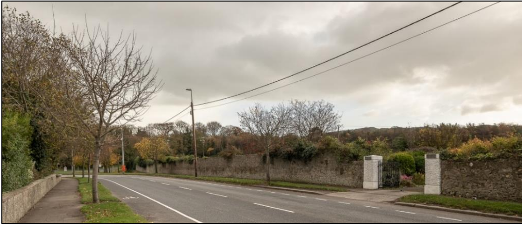
PLATE 1 NORTHERN DEMESNE WALL
